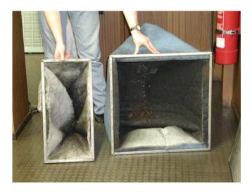
Figure 2: Bag filter, supply air filter of the HVAC installation
