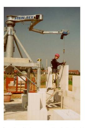
Recording of body posture and handled load weight during masonry work with the use of a mini crane as a handling aid
